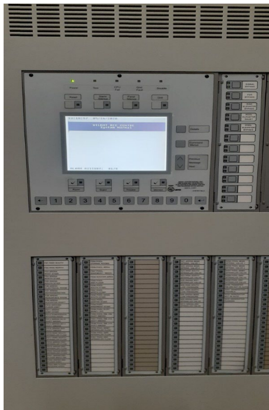
ANNUNCIATOR FIRE PANEL-MECHANICAL ROOM 1043
